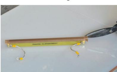
9. Cut the remaining sealing tape on the ends to allow them to fold over.
